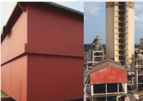
Onsite Rubber Lining
